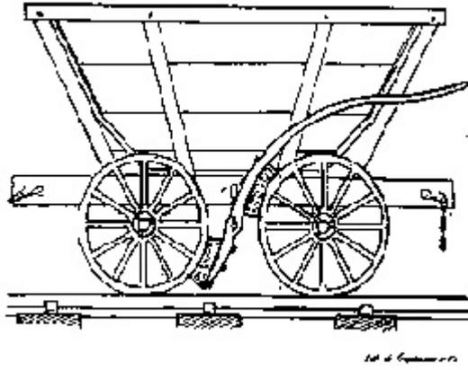
*Brake system of a wagon around 1827*
